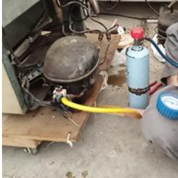
Figure VIII.- Charging R-134a Refrigerant
